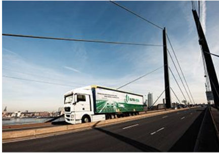
Demo trailer on bridge
