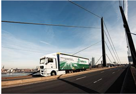
Demo trailer on bridge
